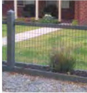
Woven wire on a timber frame
