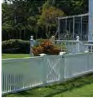
Pickets capped by a top and bottom rail
